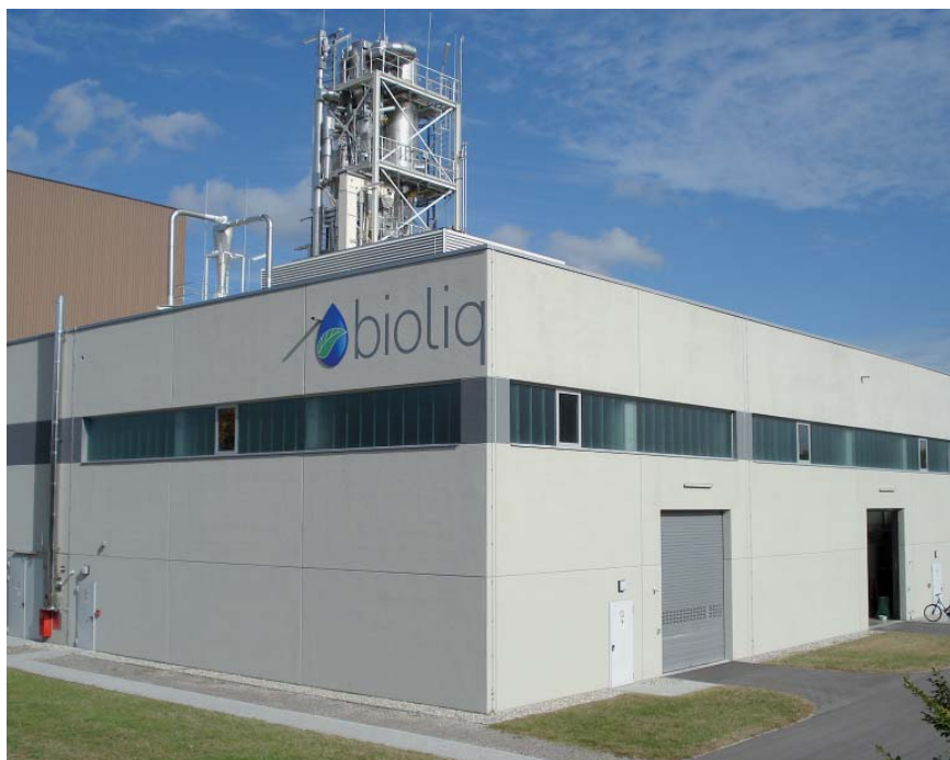
④ Process building of the pyrolysis pilot plant at the KIT
