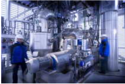
View into the bioliq® plant. (Photo by: Markus Breig)
