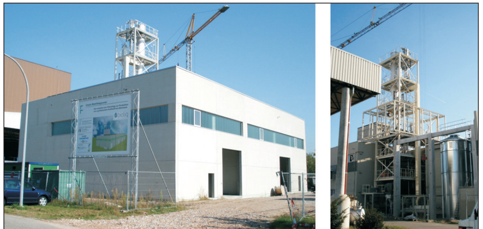
Fig. 6 Process building for biomass conditioning, fast pyrolysis and slurry preparation
